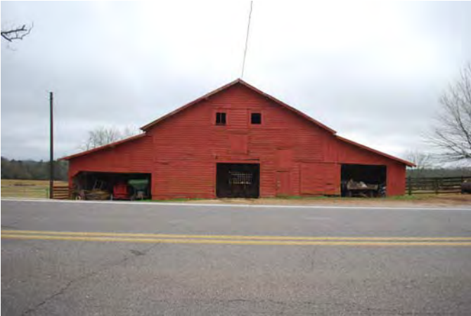
Photograph 047 Resource 14 – Frame Barn Southerly View of Front (North) Façade
