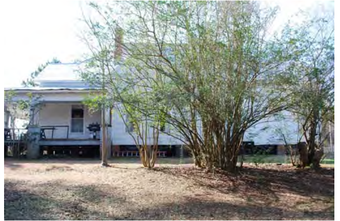
Photograph 008 Resource 1 – Main House Westerly View of East Facade
