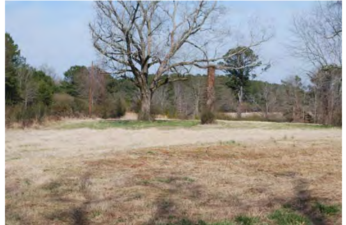
Photograph 038 Resource 6 – Historic Chimney Northeasterly View Toward Brick Chimney
