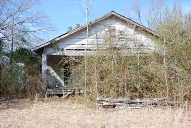
Photograph 023 Resource 2 – Secondary Dwelling Northerly View of Front (South) Facade
