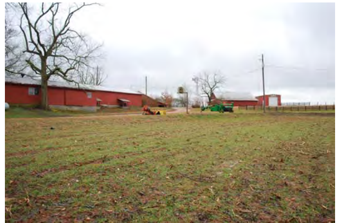
Photograph 040 Resource 8 – Gabled Shop/Garage Southwesterly View Toward Resource and Fields
