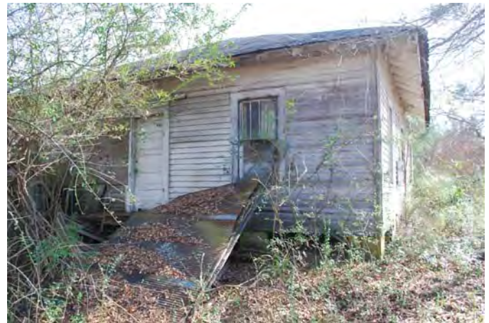
Photograph 026 Resource 2 – Secondary Dwelling Southeasterly View of Northwest Oblique
