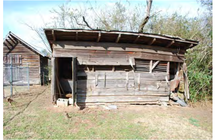
Photograph 036 Resource 5 – Frame Shed Northerly View of Front (South) Façade
