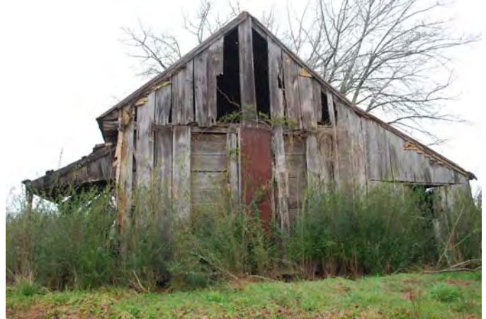
Photograph 052 Resource 16 – Sharecropper House Northeasterly View of Southwest Oblique
