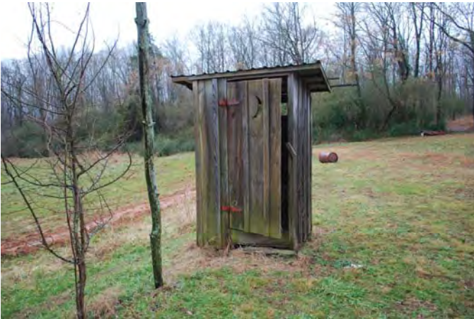
Photograph 035 Resource 7 – Outhouse Reconstruction Northerly View of Front (South) Facade
