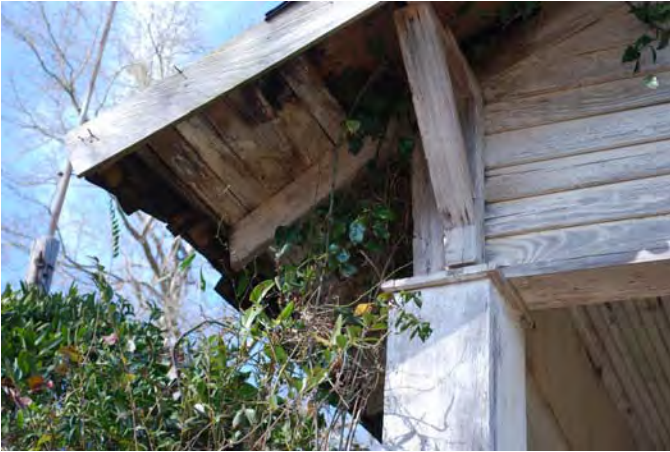
Photograph 029 Resource 2 – Secondary Dwelling Porch Gable Detail
