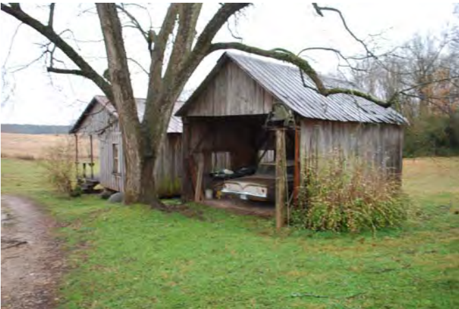
Photograph 021 Resource 4 – Frame Garage Northwesterly View of Southeast Oblique
