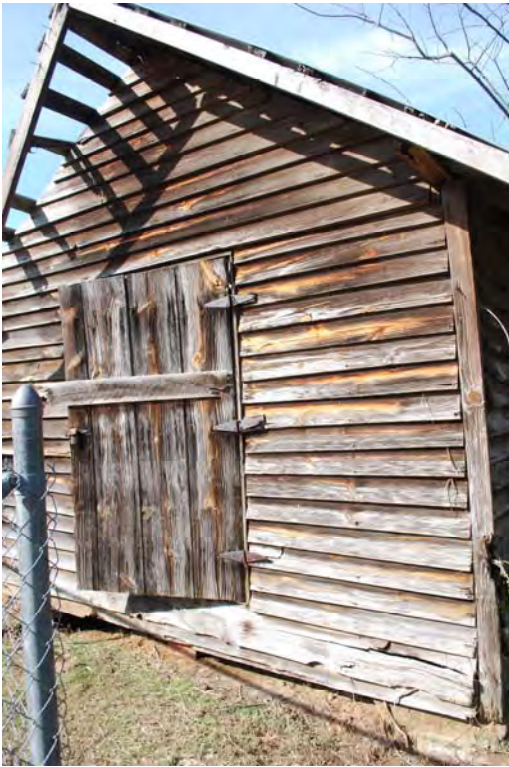
Photograph 035 Resource 4 – Frame Shed Northwesterly View of Front (South) Façade
