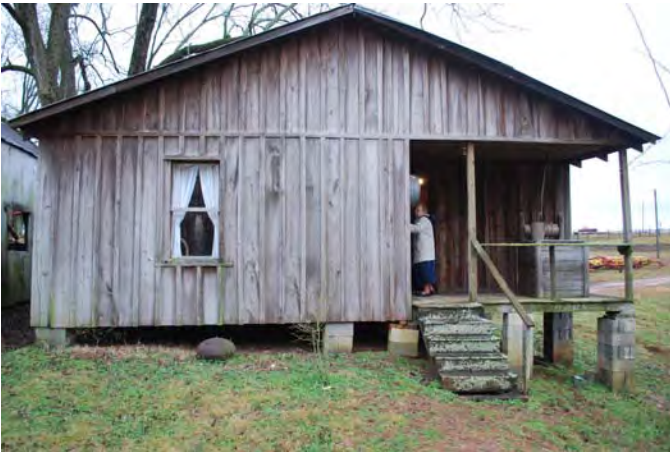
Photograph 025 Resource 6 – Early 20 th c. Cottage Reconstruction Southerly View of Rear (North) Facade
