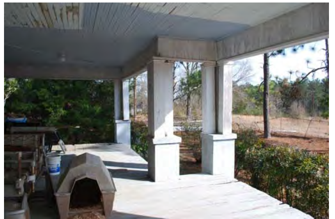
Photograph 012 Resource 1 – Main House Porch Detail
