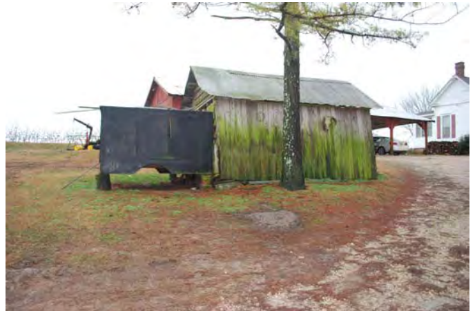
Photograph 018 Resource 4 – Frame Shed Easterly View of West Façade
