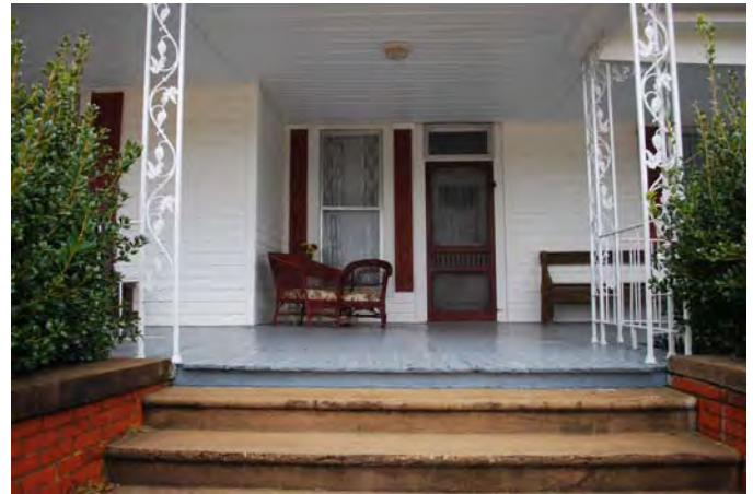
Photograph 008 Resource 1 – Main House Entry Door
