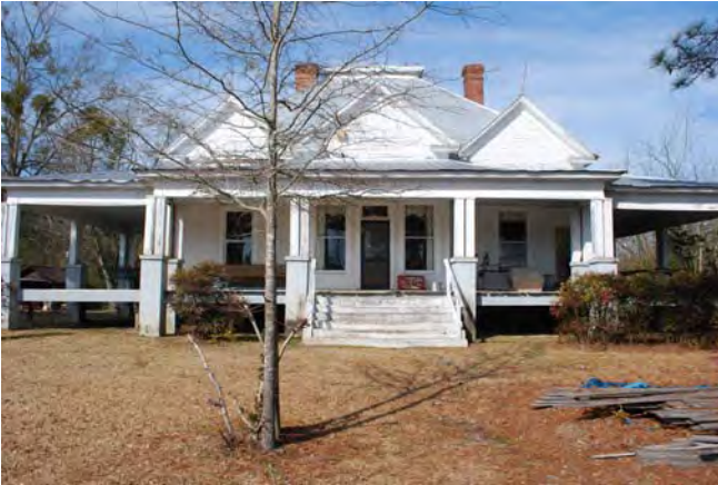
Photograph 001 Resource 1 – Main House Northerly View of Front (South) Facade
