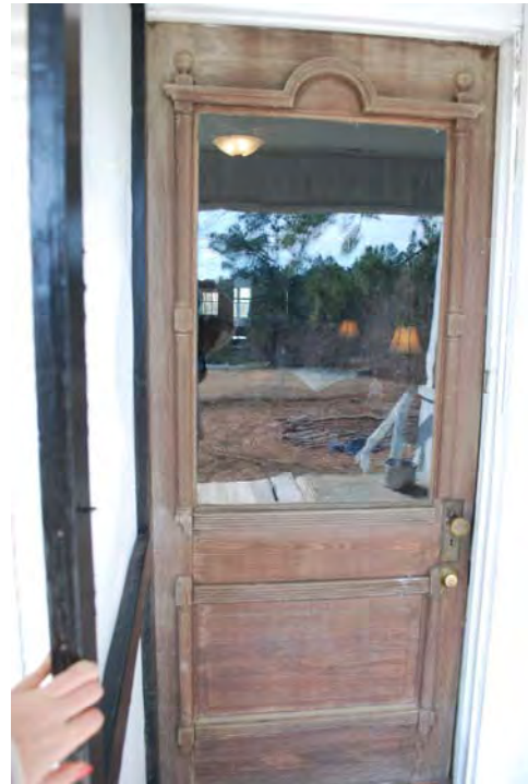
Photograph 014 Resource 1 – Main House Entry Door Detail
