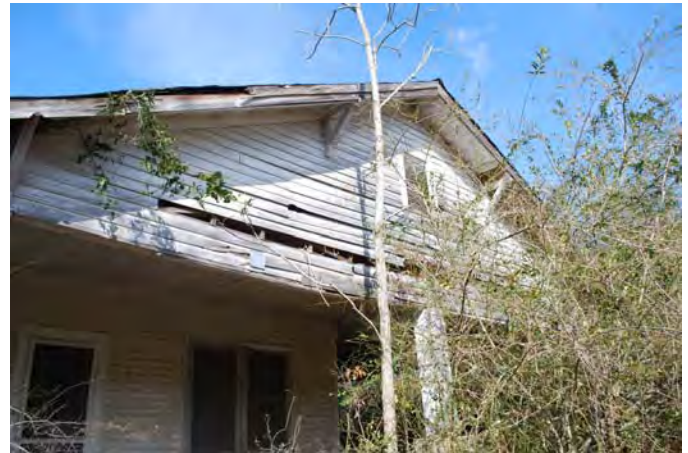
Photograph 028 Resource 2 – Secondary Dwelling Porch Gable Detail
