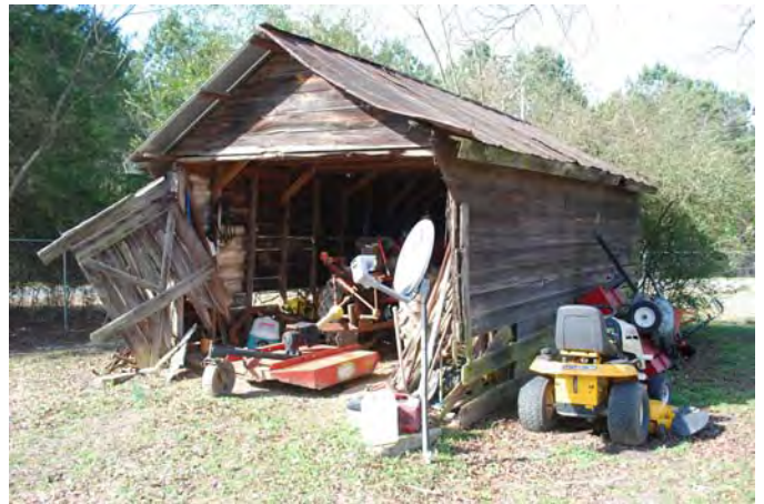
Photograph 032 Resource 3 – Frame Equipment Shed Southwesterly View of Northeast Oblique
