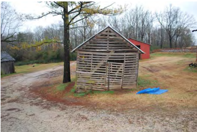
Photograph 017 Resource 4 – Frame Shed Northerly View of Front (South) Façade
