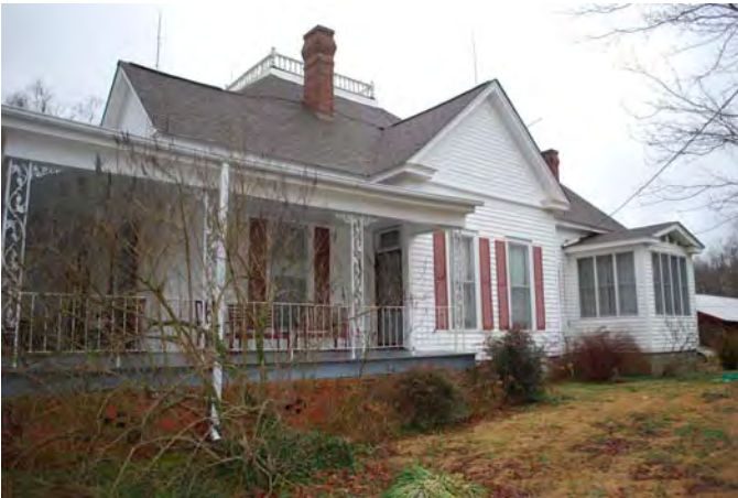
Photograph 007 Resource 1 – Main House Northwesterly View of East Façade
