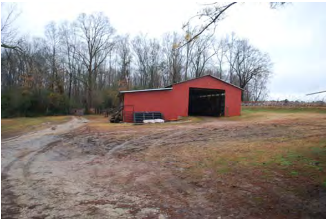
Photograph 015 Resource 3 – Equipment Shed/Garage Northerly View of Front (South) Façade
