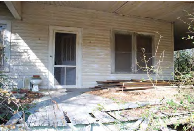
Photograph 027 Resource 2 – Secondary Dwelling Porch Detail
