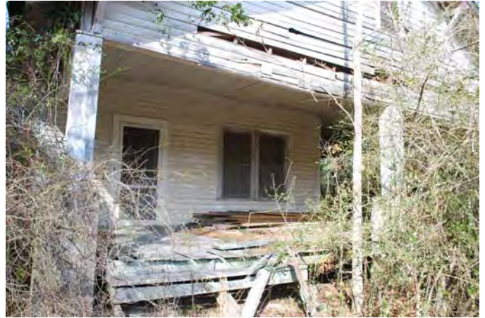
Photograph 030 Resource 2 – Secondary Dwelling Porch Detail and Condition
