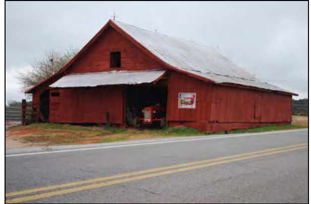
Figure 33: 2010 Photograph of Slay Farm Barn (Resource 13)
