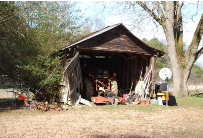
Photograph 031 Resource 3 – Frame Equipment Shed Northwesterly View of Southeast Oblique
