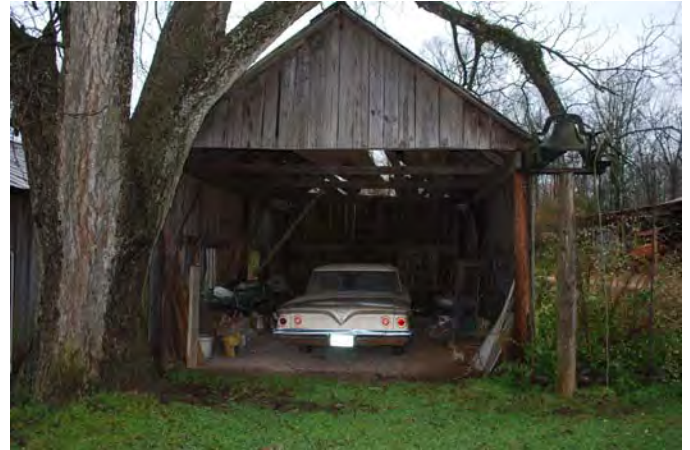
Photograph 020 Resource 5 – Frame Garage Northerly View of Front (South) Facade
