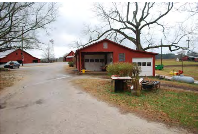
Photograph 039 Resource 8 – Gabled Shop/Garage Southwesterly View of Garage End
