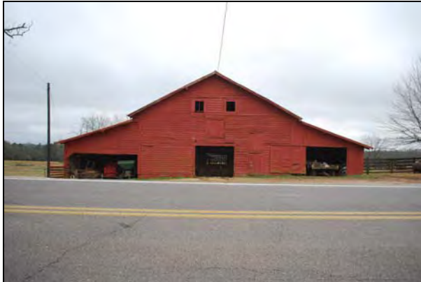
Figure 34: 2010 Photograph of Slay Farm Barn (Resource 14)
