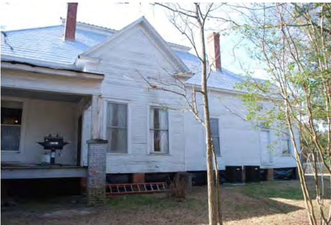
Photograph 009 Resource 1 – Main House Southwesterly View of Front Façade
