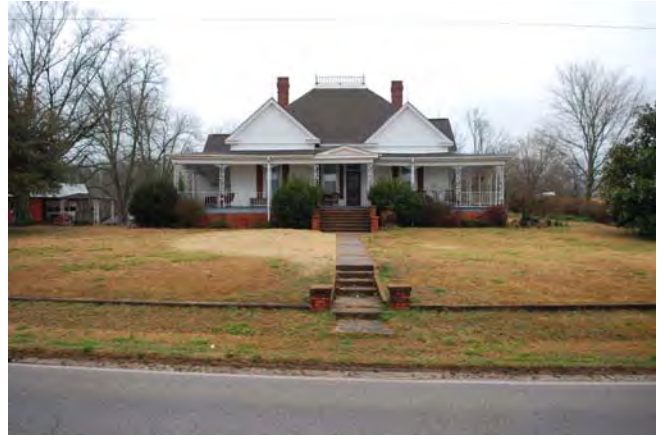
Photograph 002 Resource 1 – Main House Northerly View of Front (South) Facade
