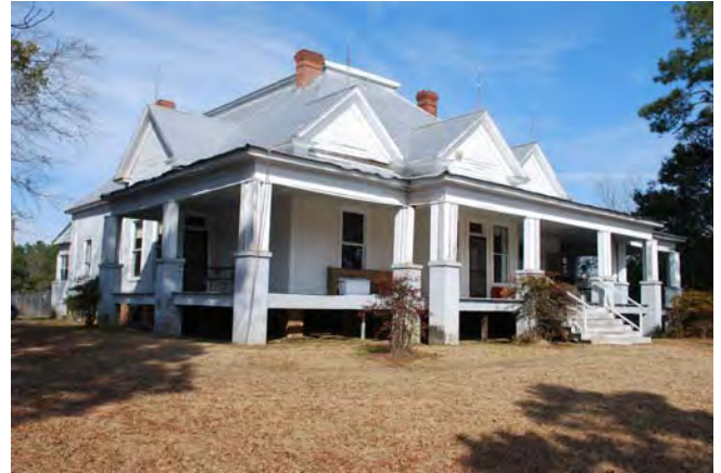
Photograph 002 Resource 1 – Main House Northeasterly View of Southwest Oblique
