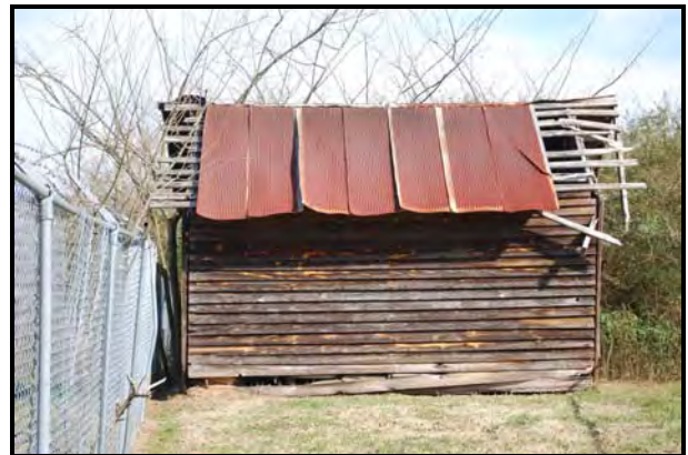
Figure 18: 2010 Photograph of Frame Shed on Holland Homestead (Resource 4)
