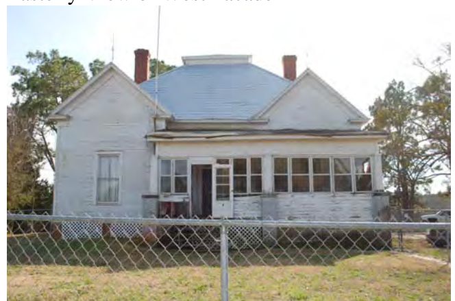
Photograph 006 Resource 1 – Main House Southerly View of Rear (North) Facade
