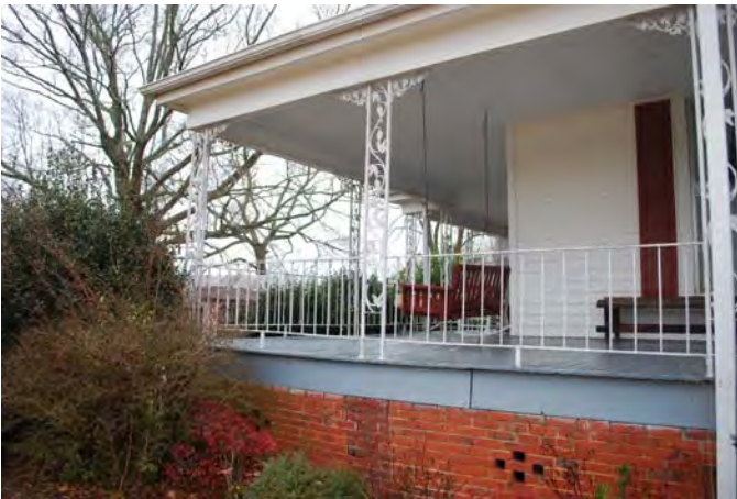
Photograph 009 Resource 1 – Main House Front Porch Detail
