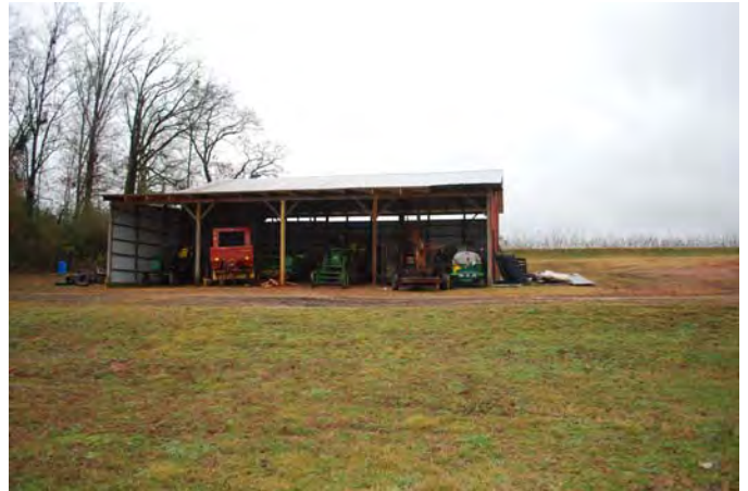
Photograph 016 Resource 3 – Equipment Shed/Garage Easterly View of West Façade
