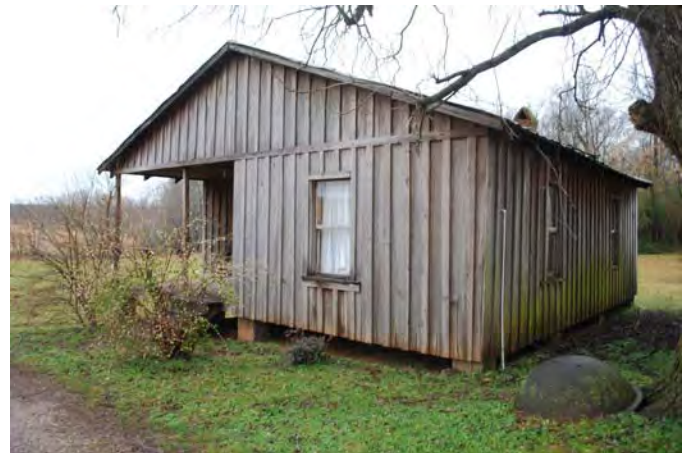
Photograph 024 Resource 6 – Early 20 th c. Cottage Reconstruction Northwesterly View of Southeast Oblique
