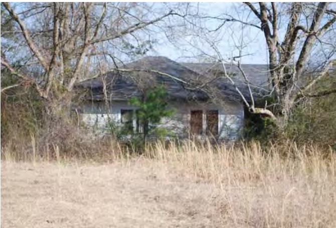
Photograph 025 Resource 2 – Secondary Dwelling Easterly View of West Facade
