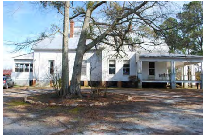
Photograph 004 Resource 1 – Main House Easterly View of West Facade
