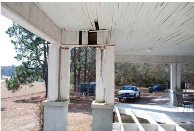
Photograph 015 Resource 1 – Main House Porch Detail
