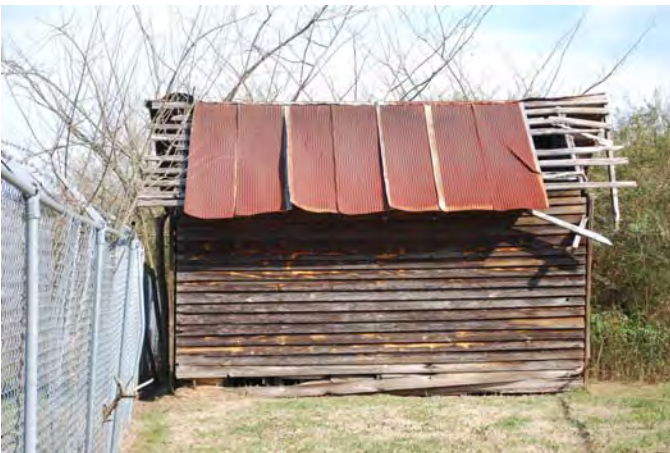
Photograph 033 Resource 4 – Frame Shed Easterly View of West Facade
