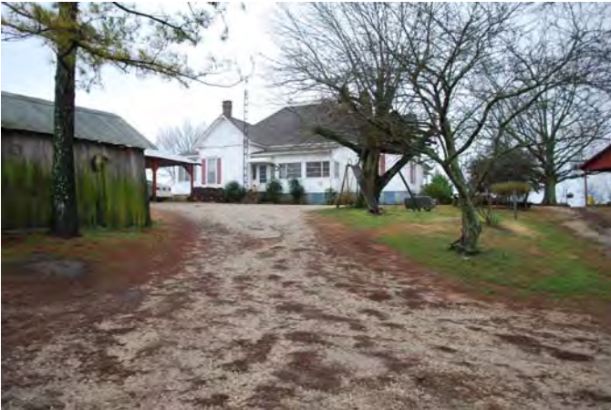
Photograph 053 Southeasterly View Toward Main House
