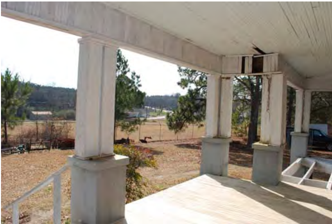
Photograph 013 Resource 1 – Main House Porch Detail
