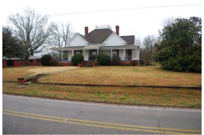
Photograph 004 Resource 1 – Main House Northwesterly View of Front (South) Facade
