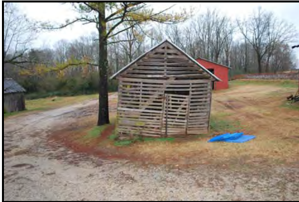
Figure 25: 2010 Photograph of Slay Farm Frame Shed/Chicken Coop (Resource 4)
